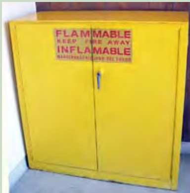
Flammable liquids storage cabinet
