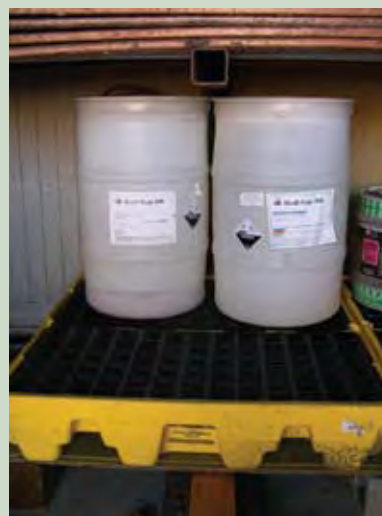
Waste containers with secondary containment
