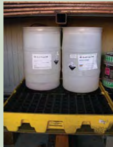
Waste containers with secondary containment
