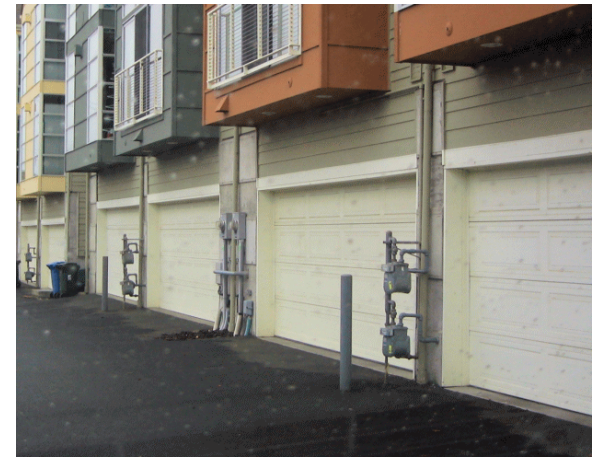
Figure F-6. Exposed utility meters like this will not be allowed.
