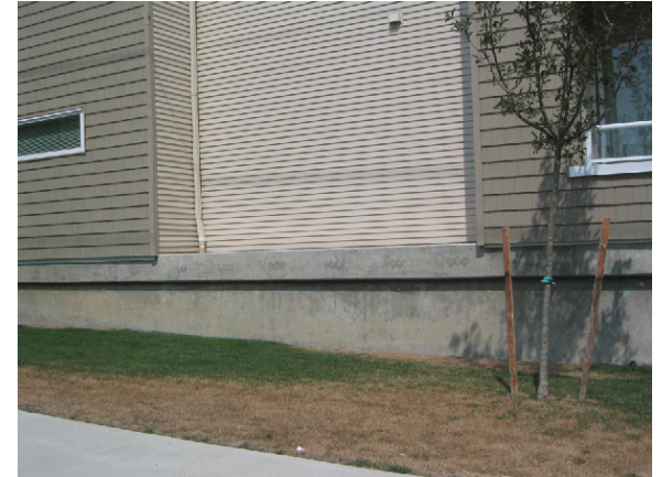
Figure F-3. Exposed foundations like this should be landscaped with shrubs and other plantings for screening.
